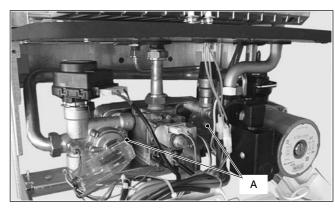
Attention. When reassembling the exchanger be sure to put the off center location/securing pin indicated towards the left side of the boiler.
